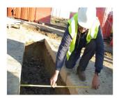
1) Measure the trench width with a measuring tape to make sure the road plate is suitable. Make sure the trench does not exceed 700mm.
