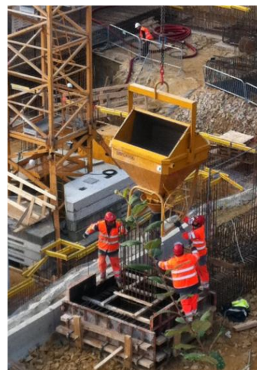
Laydown concrete skip fitted with a TE gate
